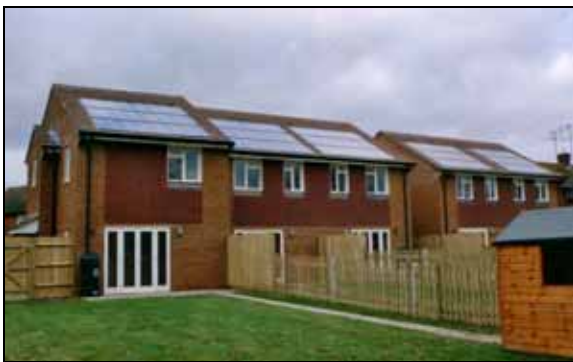
Figure 25: 5 x 1.75 kWp roof integrated PV arrays
