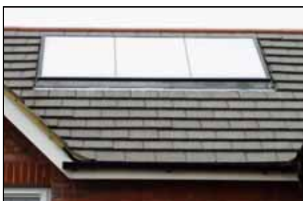
Figure 33: Integrated flat plate collector
