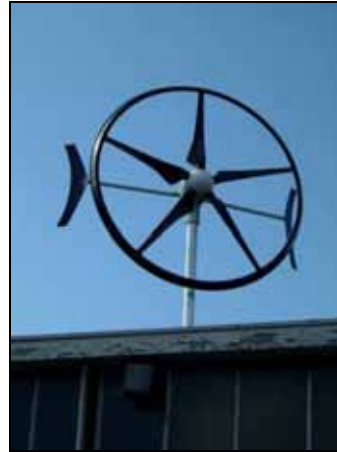
Figure 4: 1.5 kW building mounted wind turbine (2 m diameter)
