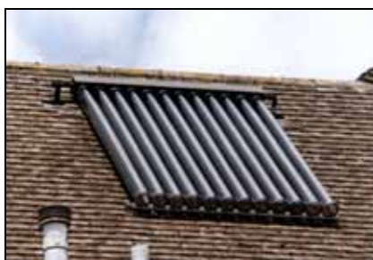
Figure 32: Evacuated tube collector
