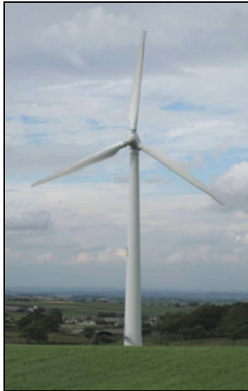
Figure 1: Large Horizontal Axis Wind Turbine (500 kW, 54m tip height) Royd Moor, Penistone.
