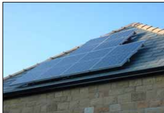
Figure 26: 0.75 kWp non-integrated PV array
