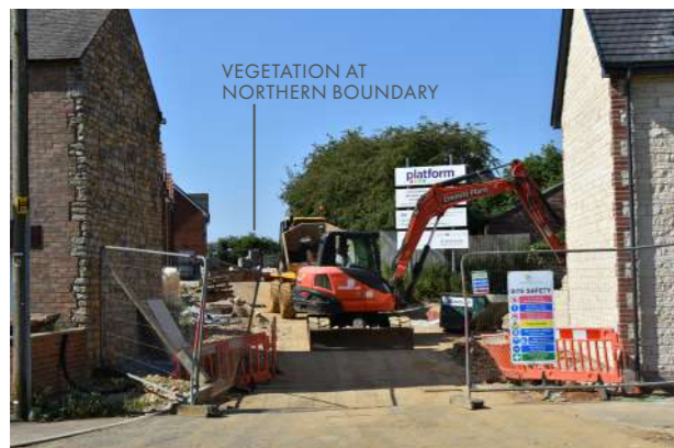
VIEWPOINT 6 LOOKING SOUTH FROM THE HIGH STREET. VIEWS OF THE SITE'S NORTHERN BOUNDARY VEGETATION ARE GLIMPSED BETWEEN BUILT FORM
