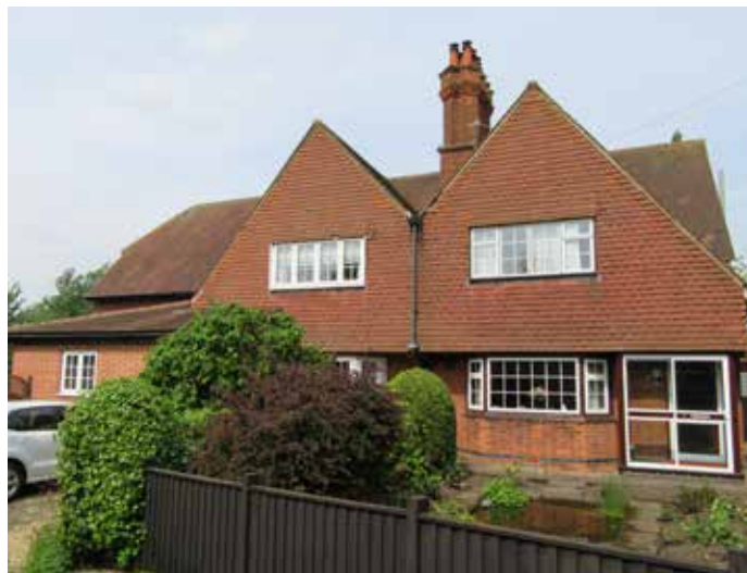
Fig 80: No.2 and 4 The Lane are characterised by their tile-fronted, low-sweeping gables, and the towering and ornate chimney stack.
