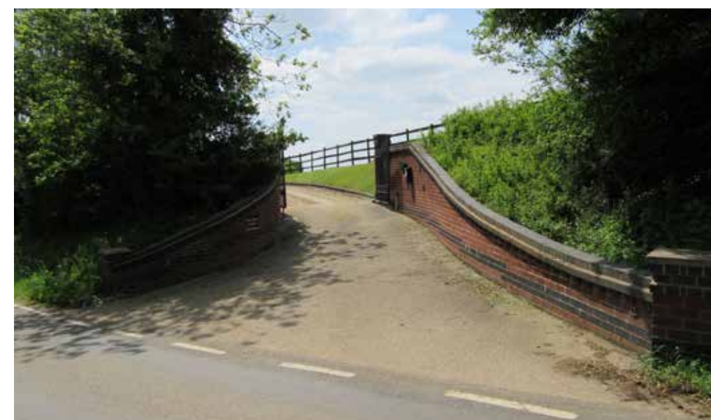
Fig 318-320: Isolated breaks in the roadside hedgerows accommodate vehicular entrances to the few properties that occupy this far northern end of Ragdale. The most respectful of the area's rustic, rural character are those accesses that tend to take a more subtle, understated approach (top image) and which minimise the break in the roadside planting and the subsequent visual impact on the approach into Ragdale.
