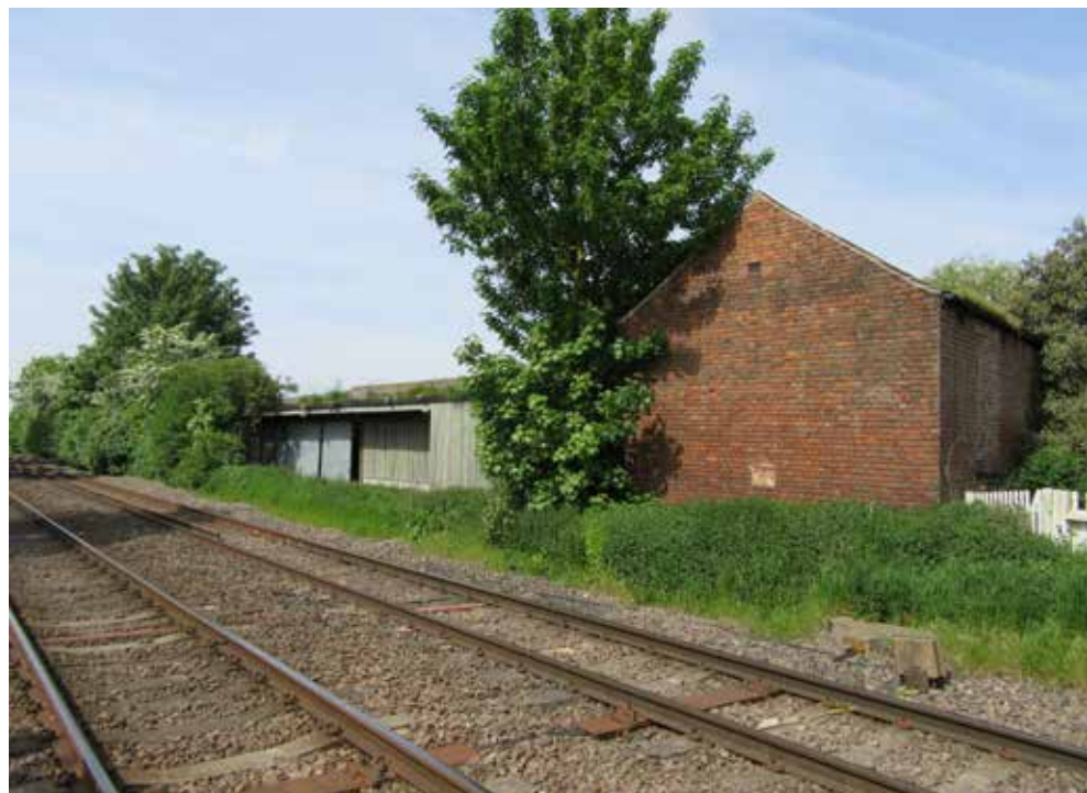
Fig 391: Present on the 1884 maps, this red brick building was likely part of the original railway station complex. Today it stands prominently along Hoby Road and forms part of the Wreakside Centre.
