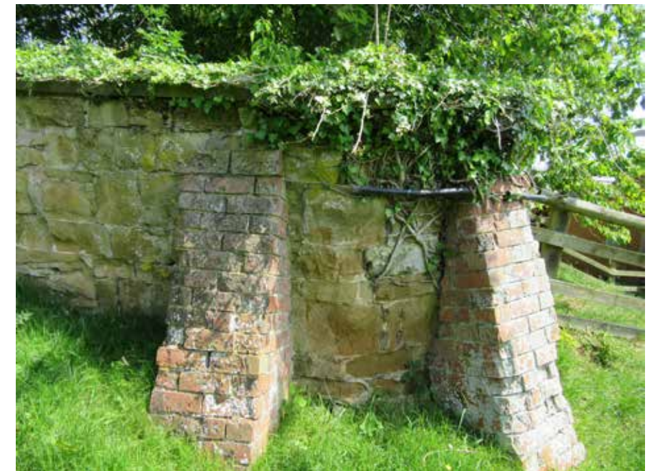
Fig 309 and 310: Enclosing the churchyard and enhancing the church setting is a handsome boundary wall of coursed, squared ironstone and coursed limestone rubble with grey sandstone coping.
