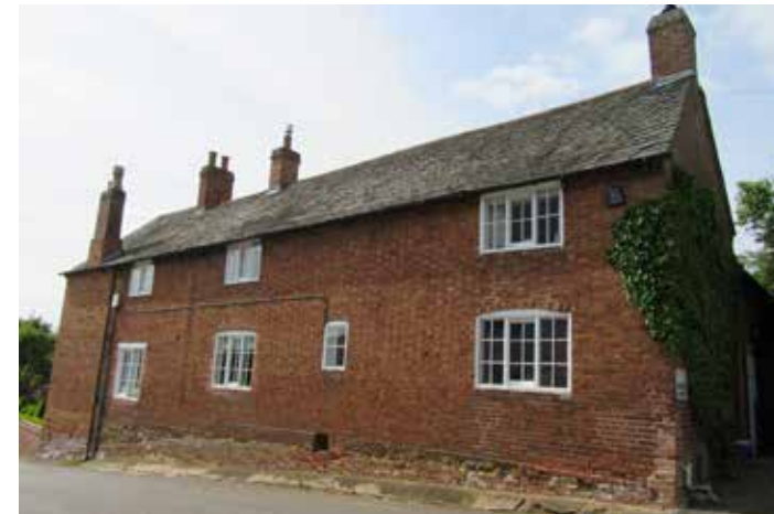
Fig 140: Built in 1774, Glebe Farmhouse (Grade II) is an imposing two-storey dwelling that stands confidently at the corner of Main Street and Thrussington Road. It is constructed of red brick in Flemish bond and topped with a pitched Swithland slate roof that accommodates several chimney stacks.
