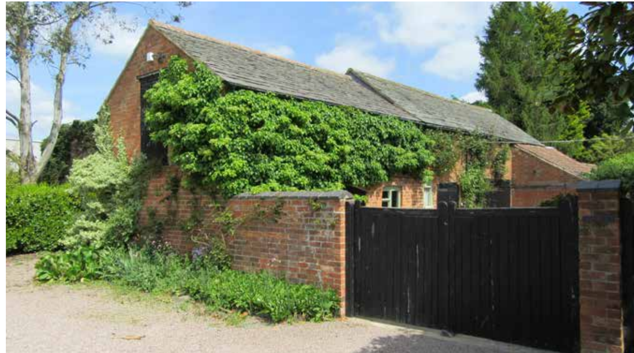
Fig 275: An important local building in its own right, the large 19th century outbuilding at Home Farm, which runs perpendicular to Main Street, is a handsome vernacular structure and one of Ragdale's best preserved traditional agricultural buildings.
