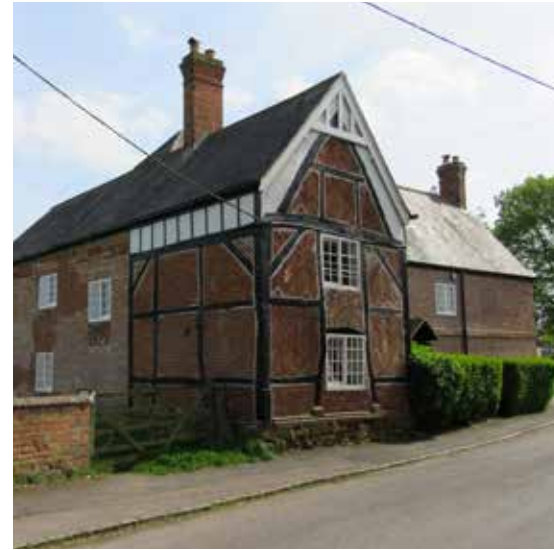
Fig 136: The Homestead (Grade II listed) is a 17th century farmhouse with 18th and 19th century additions. Of red brick with ironstone plinth and slate roof, the building has a particularly noteworthy older timber-framed wing, which extends out to the street, and accommodates brick infills with a herringbone pattern.
