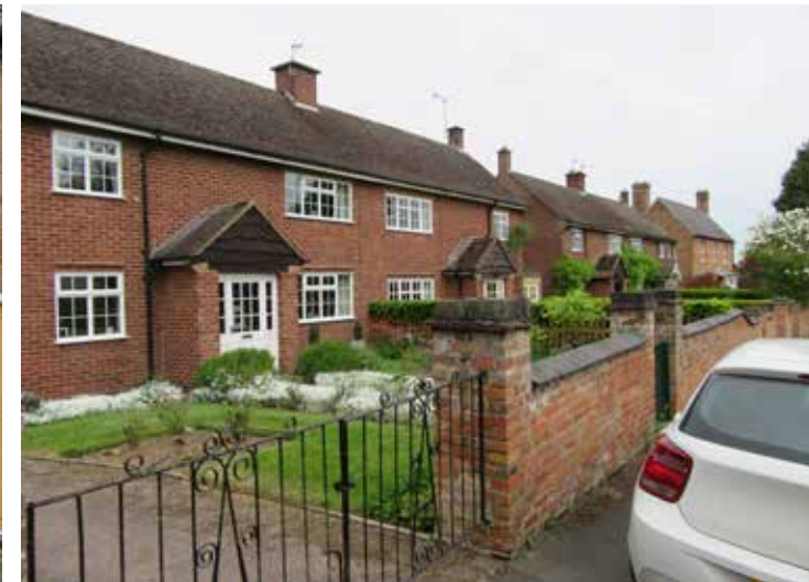
Fig 78: No.17, 19, 21, and 23 Main Street form a strong frontage along the central part of Main Street, their unpretentious semi-detached, two-storey forms adhering to a common building line and the same uniform design and detailing.
