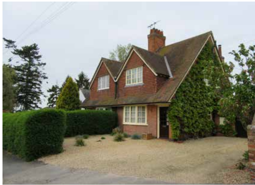
Fig 73: No.3 and 5 Main Street are a charming pair of semi-detached inter-war properties with distinctive red tile clad dormers projecting from their steep and tall pitched roofs and a centrally positioned, shared chimney stack. Timber framed bay windows feature at ground floor level, whilst at first floor casement windows are present.
