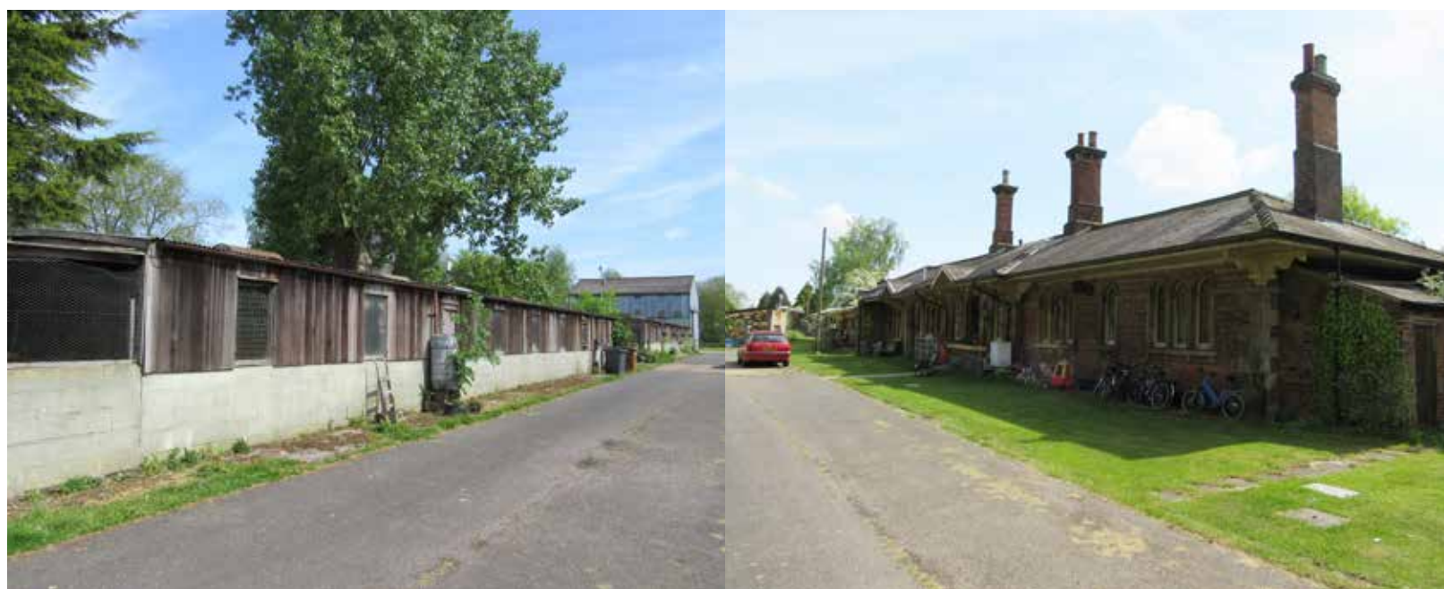
Fig 347: The former Brooksby Station building, now in residential use, stands at the northern entrance into Brooksby.
