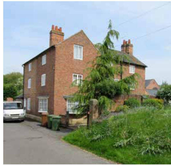
Fig 72: Formerly a post office, farmhouse and dwelling, these buildings now comprise a pair of houses. Grouped under a single listing (Grade II), Laburnum House and Post Office Farmhouse display a sizeable three-storey form of red brick with pitched slate roofs accommodating brick ridge stacks.
