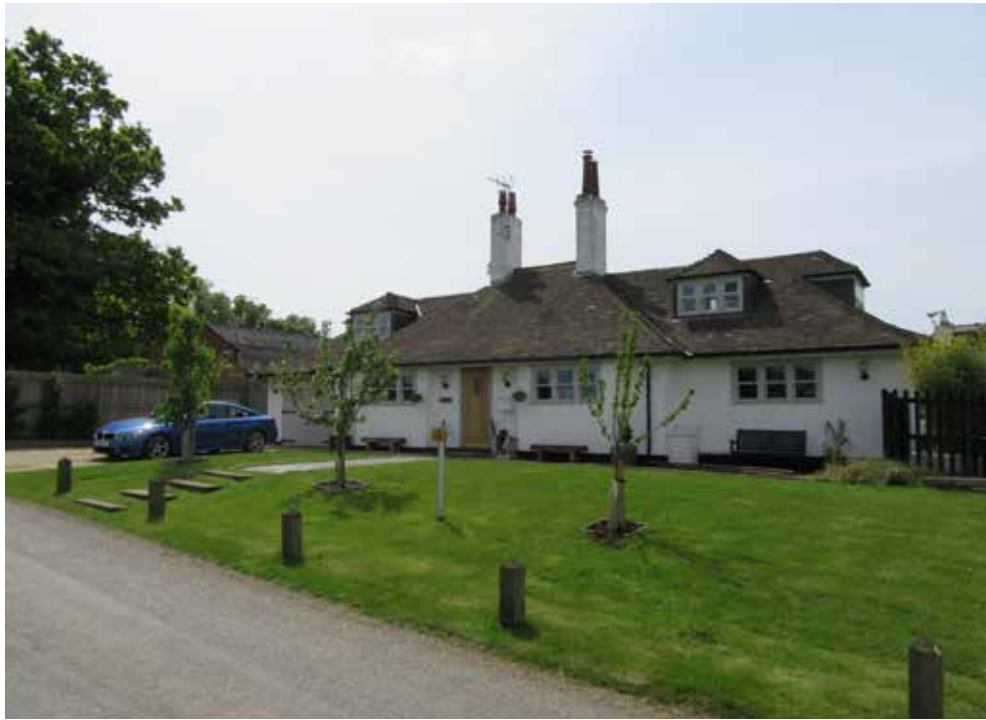
Fig 398: Brooksby Lodge, first appearing on the 1953 map, has been extended and altered in recent years. However, the two tall chimney stacks, which were a defining feature of the original building remain perched along the ridge of its hipped roof, and the extension works have been carried out in a sensitive manner, resulting in a modern home of charm and character.
