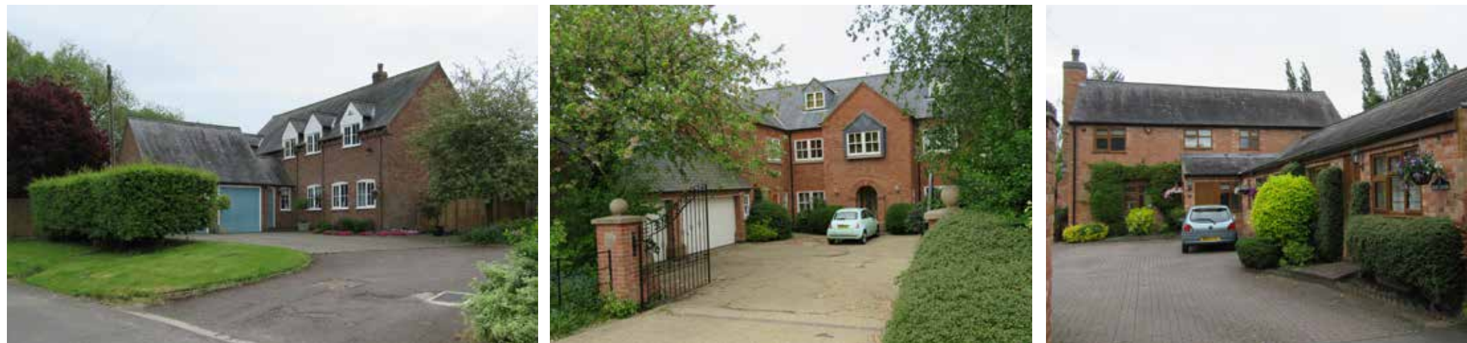
Fig 84-86: The majority of Rotherby's more recent additions to the village townscape have adopted a materials palette of red brick with slate roofing, which responds positively to the local character and helps these modern buildings integrate into the village setting.
