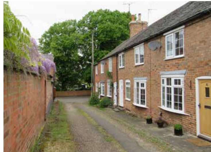
Fig 77: The Row comprises a single terrace of traditional red brick cottages, several with Swithland slate roofs. Bay windows feature at ground floor level, with casement windows on the upper floors. Chimneys along the ridge give the roof a distinct and rhythmic profile.
