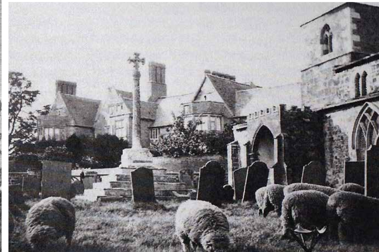
Fig 241 and 242: Old Ragdale Hall once stood alongside All Saints Church to form a particularly unique and majestic village centre. However, though today the church still stands proudly at the very heart of the village, Old Ragdale Hall was demolished in the 1950s.
