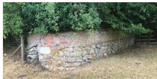
Fig 312 and 313: Forming the north edge of the paddock is the original boundary walling of the Old Hall, which is both of historic significance to the village and forms an attractive edge to this key green space.
