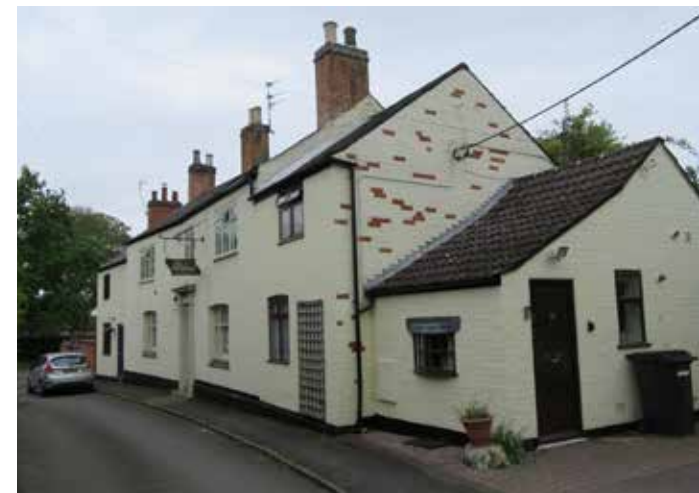
Fig 161: The Old Rutland forms a strong and distinct frontage along a significant stretch of the northern side of Regent Road. Formerly a public house (the Rutland Arms), the building is now a private dwelling. The main body of the house is rendered, with only the chimneys still displaying the original red brickwork. The traditional hanging sign mounted on the upper facade is a memorable feature that subtly hints at this property's previous life as a public house.
