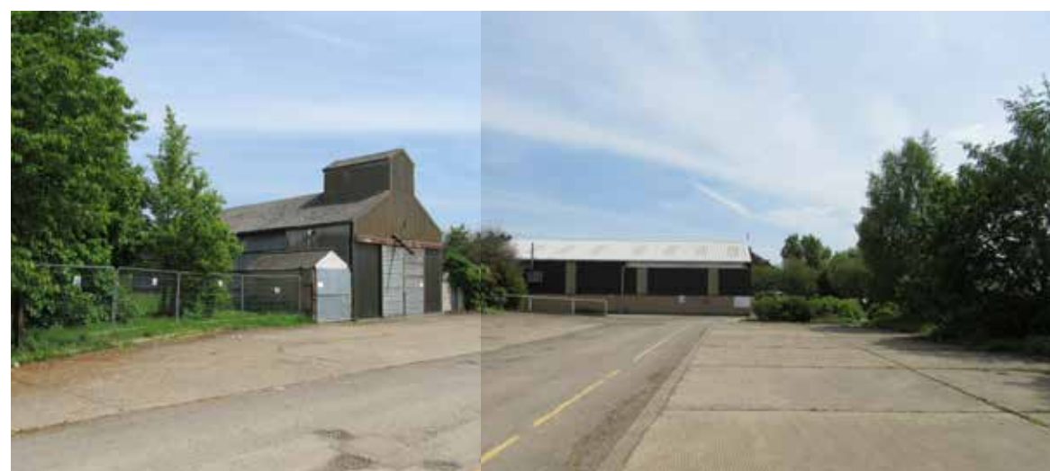
Fig 353: The Spinney Campus, which is now largely derelict, was first developed in the 1950s and has been added to and altered over subsequent decades, giving it a somewhat disorderly layout, with buildings of differing sizes and scales spread across its extents with no obvious overriding approach to positioning or orientation.
