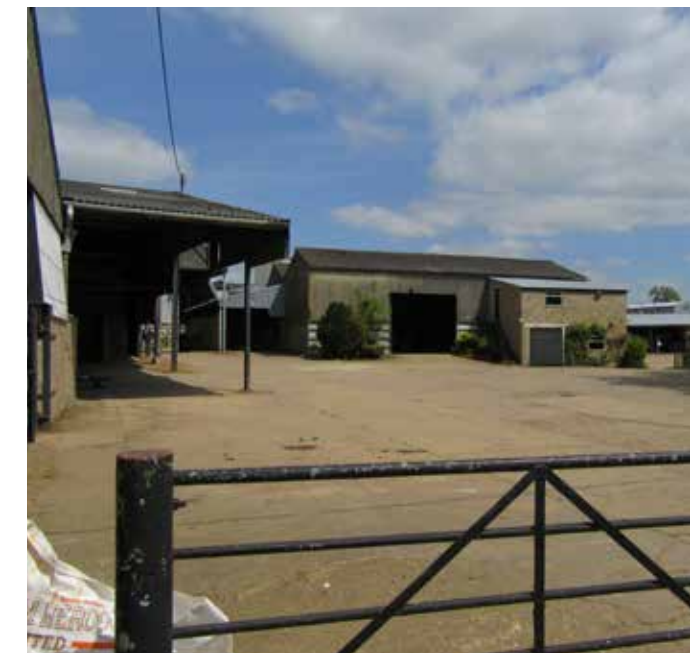
Fig 249: Extending east from Six Hills Road across an expansive site accommodating numerous large agricultural units and several smaller, vernacular outbuildings is Old Hall Farm.
