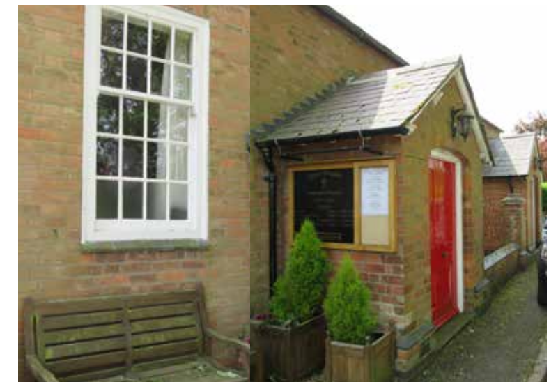
Fig 168: The 19th century Methodist Chapel forms a local landmark at the top of Chapel Lane. Its modest and understated scale and aesthetic is enlivened by two small gabled entrances with slate roofs that extend out from the main facade, each incorporating a wall-mounted lantern above painted timber doors. Two large 8-over-12 vertical sliding sash windows animate the remainder of the frontage.
