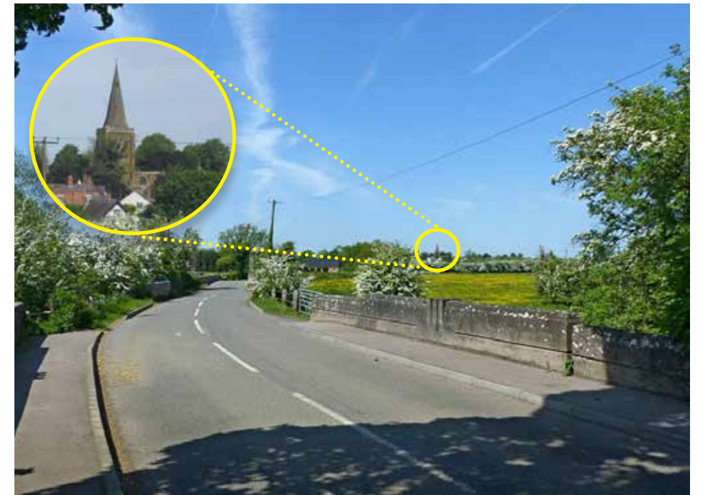
Fig 393: Constructed by Leicestershire County Council in 1935, the art deco influenced bridge at the northern gateway to Brooksby forms a handsome and distinct crossing over the River Wreake. From this position, a beautiful view towards Hoby can be gained.
