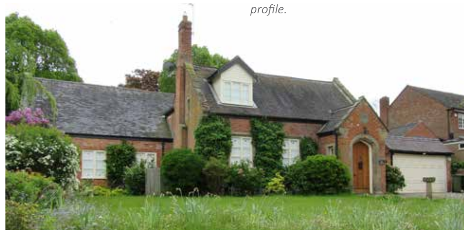
Fig 81: Constructed in 1848, the Old School House is a local landmark building and one of the village's most distinct historic buildings. Though the subject of some personalisation and extension works, the building retains much of its original character and charm, including the gabled porch that incorporates an inset stone inscription denoting the year of construction, and the stone arch doorway.
