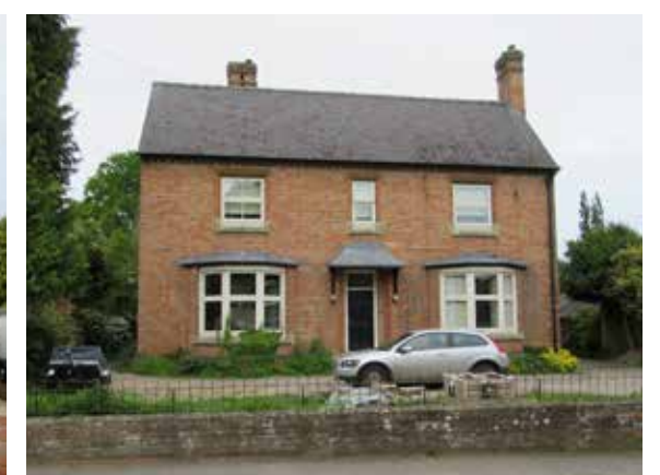
Fig 83: Manor Farmhouse is a large three-storey dwelling of red brick with slate roofing. Its side profile is a prominent feature along The Lane, whilst its 3-bay principal elevation faces on to Main Street, and accommodates a distinct central canopy over its front entrance.
