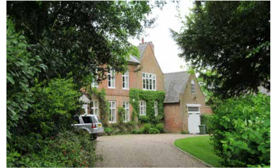
Fig 138: Tucked away in secluded, heavily-wooded gardens is the Grade II listed Old Rectory, which dates from 1703. Of red brick in Flemish bond with Swithland slate hipped roof, the Old Rectory has a restrained, formal character, displaying a strong degree of symmetry in its plan and facade arrangement, with a centrally positioned, pedimented entrance door flanked on either side by tall sash windows.
