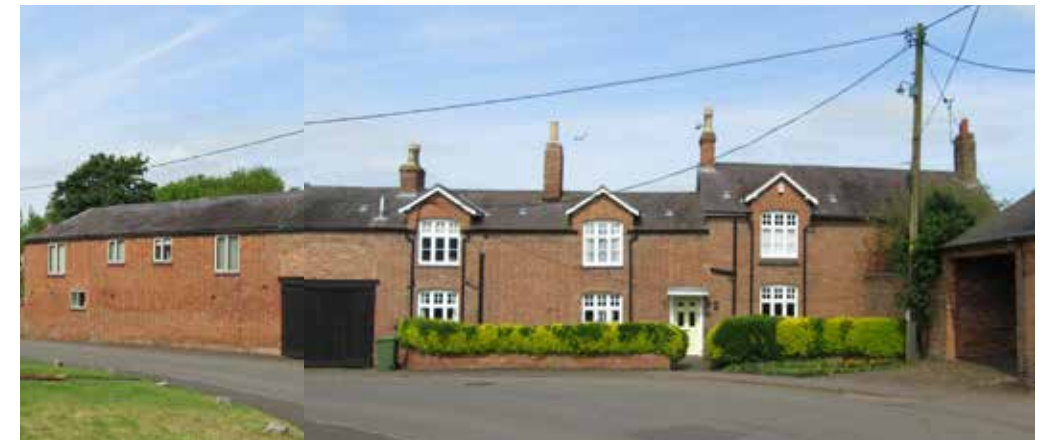
Fig 148: Gables Farm is a long, linear property, whose extensive red brick facade forms a visual stop on the bend leading out of the village at its northern end. Set to the right of the central vehicular access, the original dwelling seeks to bring a more vertical emphasis to its form through the progression of tall, slender chimney stacks and ground and first floor windows aligned below dormers.
