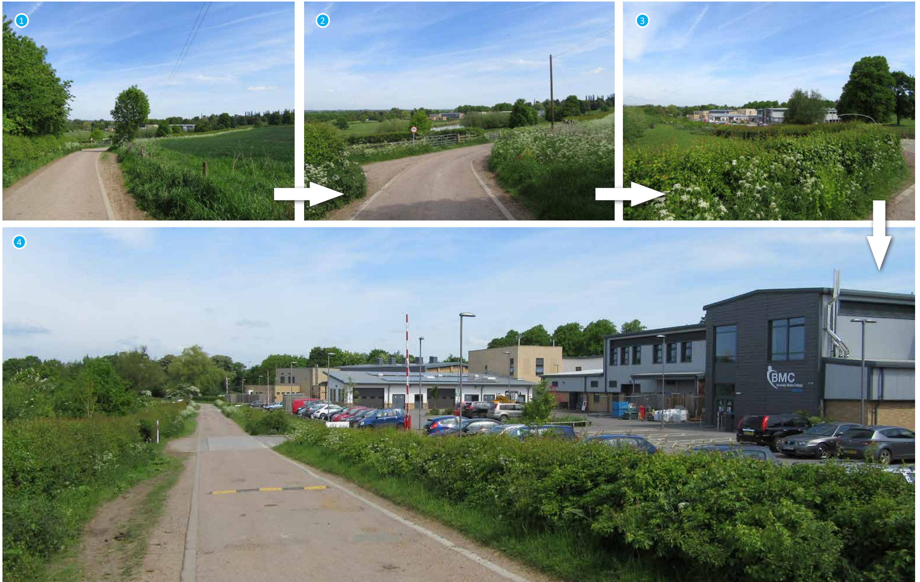
Fig 23-26: The recently constructed Brooksby Melton College buildings, located to the west of the campus core, represent the only significant incident within the parish where development has failed to respond positively to its landscape setting, with these rather substantial structures sitting quite exposed and appearing abruptly when approached from the south.
