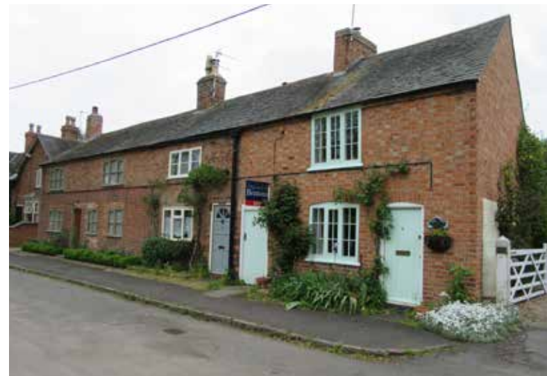
Fig 166: No.4, 6 and 8 Church Lane are a row of 19th century terraced cottages of polite design whose long, linear form projects a strong frontage on to Church Lane. Despite some personalisation across the properties, including adaptations to the original fenestration, the cottages still retain much of their original charm and character, remaining a coherent and attractive grouping.
