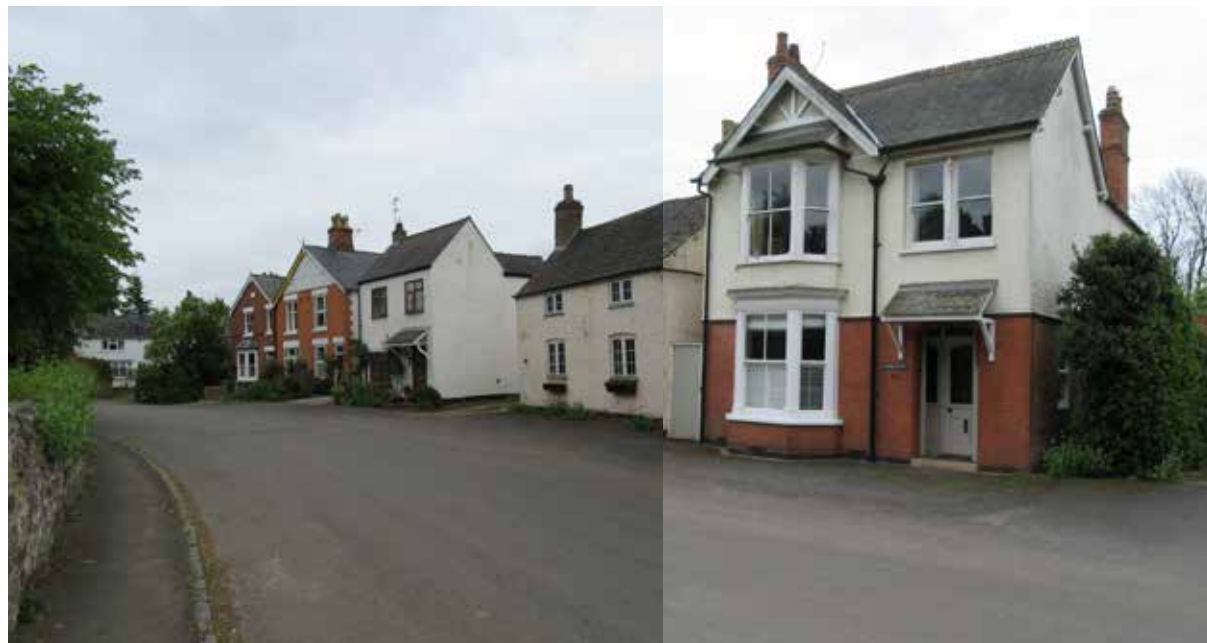
Fig 160: No.14-24 (even) Main Street are an important building grouping within the wider setting of All Saints Church, where they stand along a common building line and combine to present a strong, characterful frontage to this part of Main Street.
