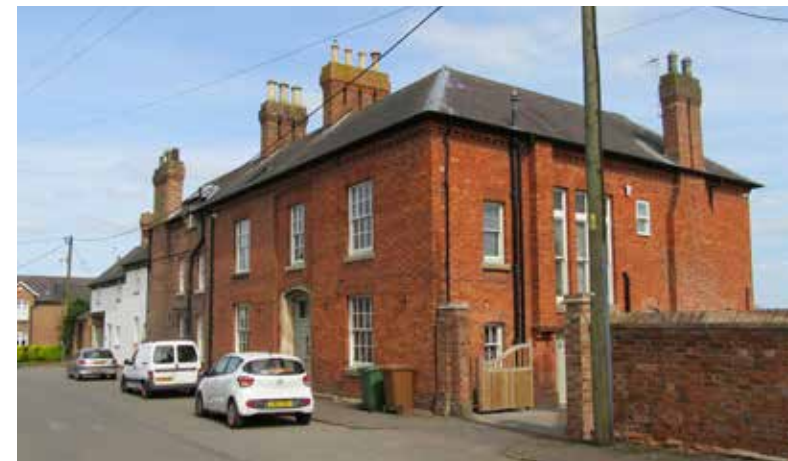
Fig 150: The Grange is a large, mid-1800s house and landmark building at the northern end of Main Street. Its bright red brick facade hosts regularly arranged sash windows (both 6-over-6 and 8-over-8) and a panelled front door enclosed by impressive stone surround, whilst imposing chimneys top the building.
