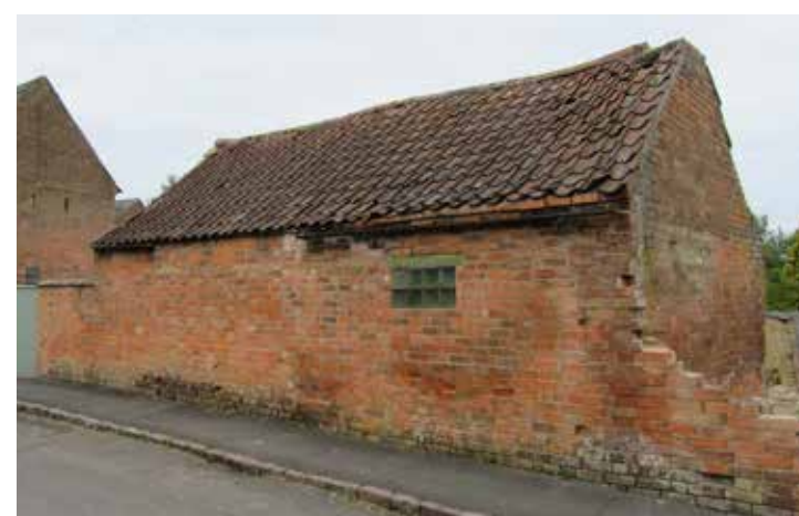
Fig 82: The small outbuilding at Orchard House currently stands in a slightly dilapidated and neglected state. Nevertheless, the building's distinct vernacular aesthetic coupled with its prominent positioning along Main Street make a locally valued building that contributes positively to the village townscape.
