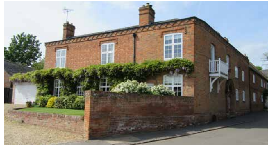
Fig 147: The Chantry is one of the most attractive and beautifully detailed buildings in the village, its stunning southern elevation with brick dentil course and thick band of wisteria greeting visitors entering the village from Brooksby Road.
