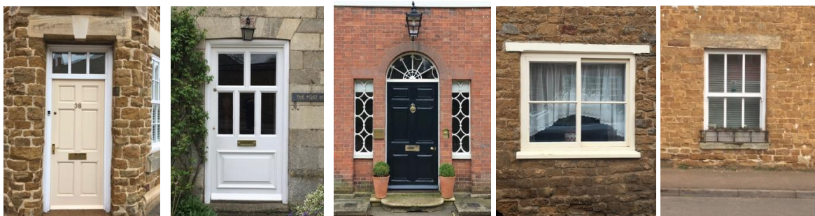
Local doors, fanlights, canopies and windows.
