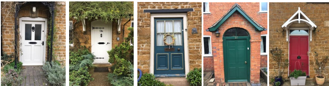
Local doors, fanlights, canopies and porches.
