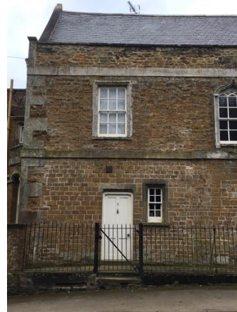
Mix of ironstone walls, red brick walls, dressed stone mullions, bays, slate roofs and string courses (High Street, Somerby).
