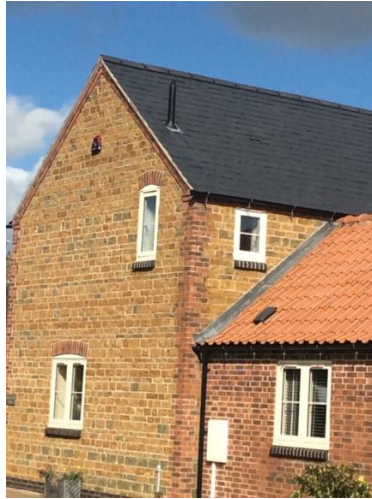
Left: Example of brick quoins framing ironstone walls (Manor lane, Somerby)
