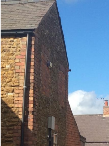
Left: Example of brick quoins framing ironstone walls (Manor lane, Somerby)
