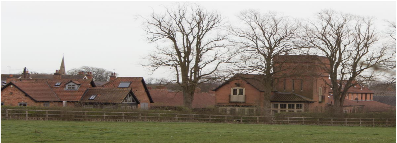
Figure 29: Grove Stables and water tower buildings at right, Burrough Road, Somerby (Map Ref 25)
