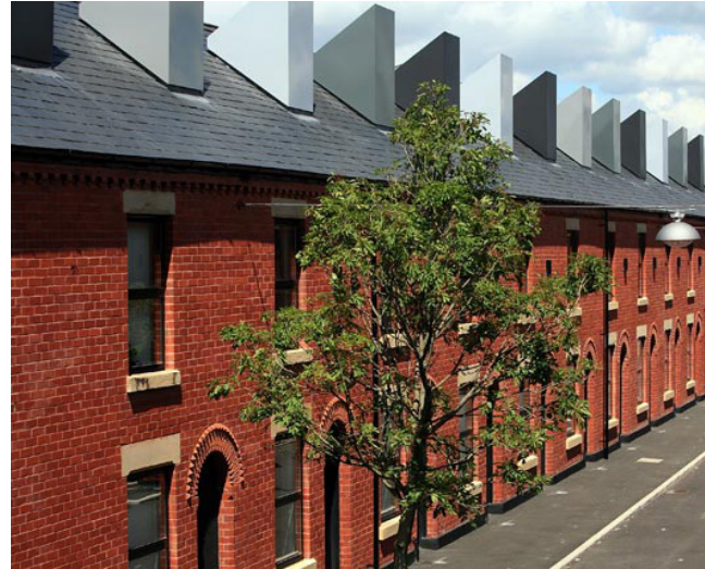
Examples of built form and architecture
